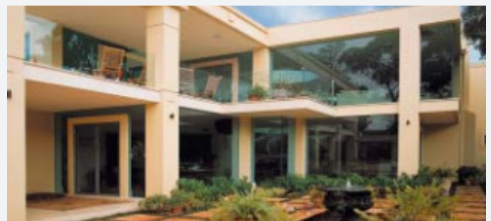
Fig 2 : Five-year old residence in Melbourne exemplifies projects in which laminated glass containing B14 PVB have exhibited no edge delamination.
